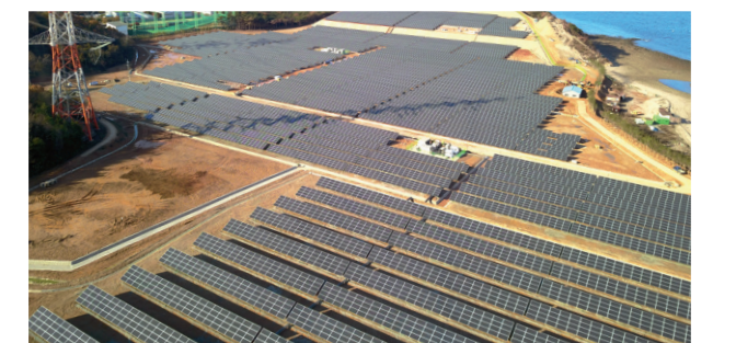
Solar farm in Dangjin
