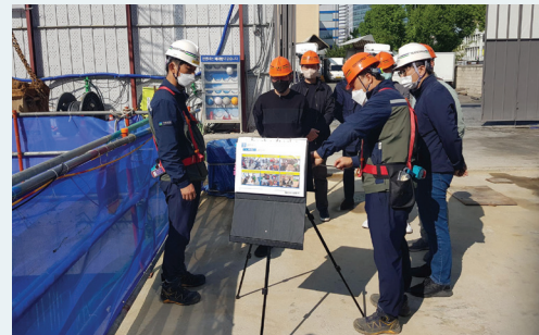
On-site safety inspection
